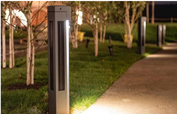
Illuminated bollard for wayfinding and safety reasons
