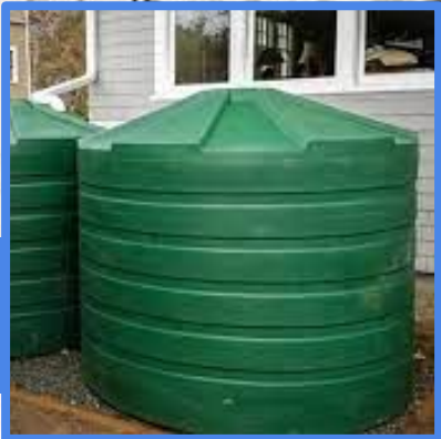
Storage Cistern (10'x10' - 6,300 Gal)
